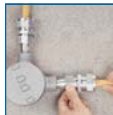
Insert assembly and tighten adaptor nut
