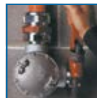
5. Install hub on enclosure
