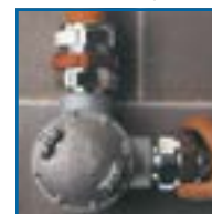
6. Insert cable and tighten red union
