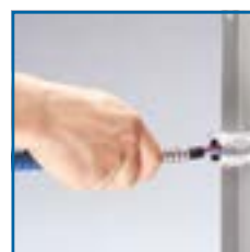
Slacken gland nut and insert prepared cable
