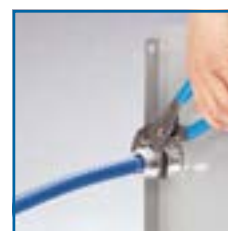
Hand tighten gland nut to hold cable, then wrench tighten
