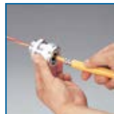
Install TCAX fitting on cable
