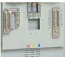
Earth and neutral bars positioned for easier cabling
