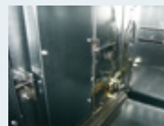
Interlock for circuit breaker compartment door
